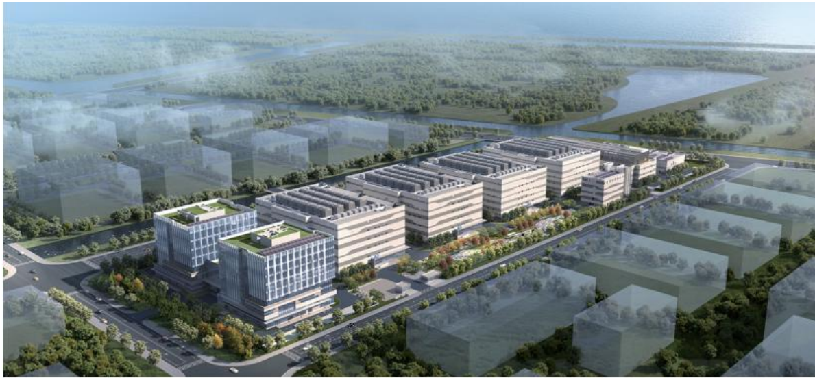
Fig.2 The design of China telecom's Lingang data center i
